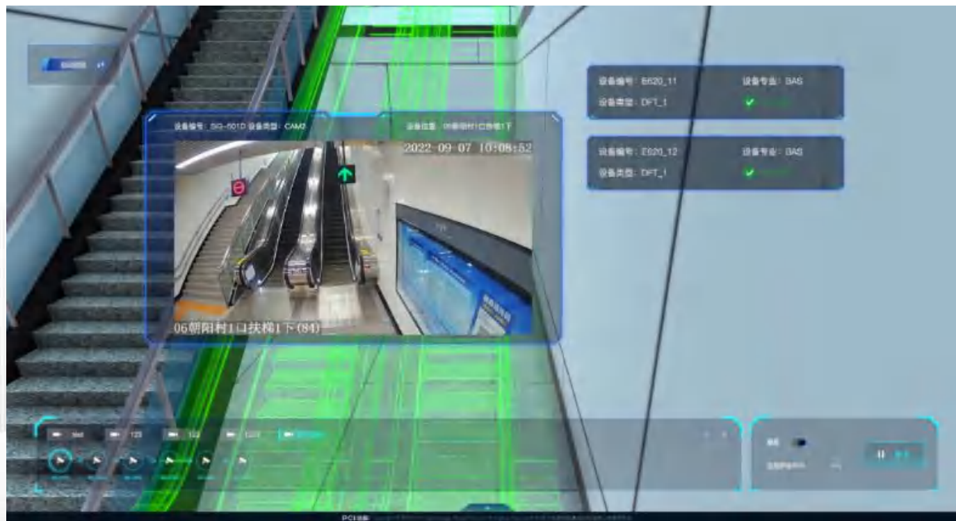
③ Video Inspection
